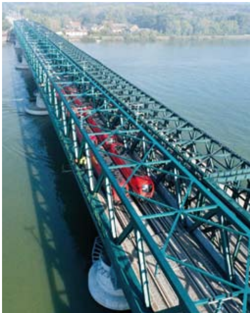
Tulln Danube Bridge
