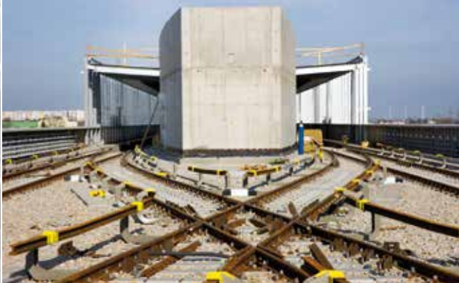
Extension of the U2 underground line, Vienna
