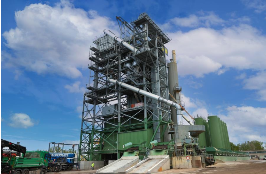
New asphalt mix plant will ensure lower carbon footprint © PORR
