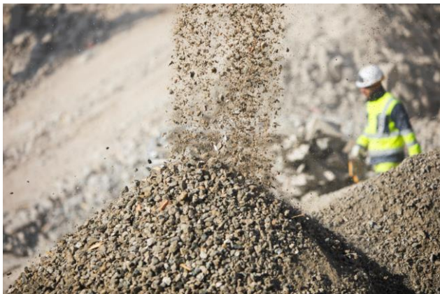
From left: A new processing plant effectively handles mineral wool © PORR Bricks get a new lease of life in the Himberg Recycling Center © PORR Concrete becomes recycled concrete © PORR
